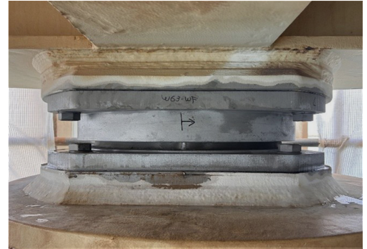
Wharf bearing assembly
